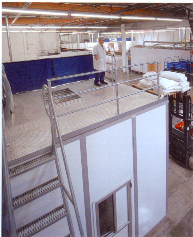
Bags of raw material forklifted to the mezzanine level are manually dumped through a screen (left of operator) into a rotary batch mixer located in the room below, in compliance with US FDA's Good Manufacturing Practices.
